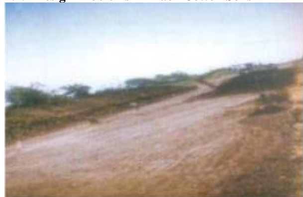
Fig. 1.2 Construction of Road Embankment with Cohesive Non Swelling Soil (Moorum)
