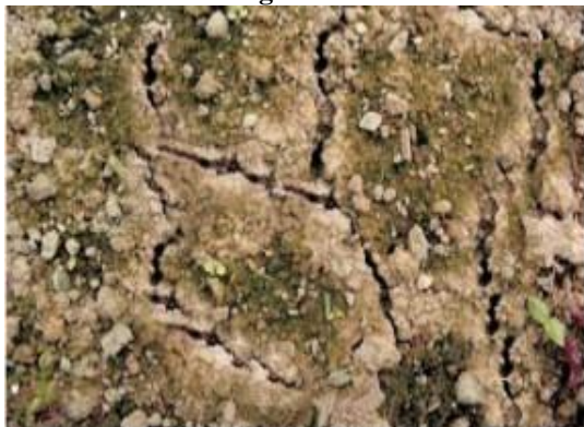
Fig. 1.1 Typical Cracks in Black Cotton Soil in Dried State
