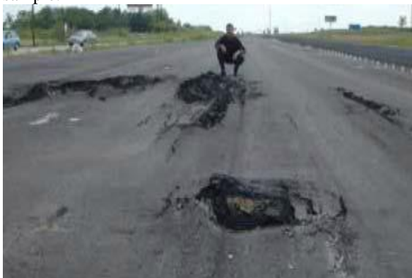
Fig. 1.3: Extreme example of pavement failure from unstable soils
